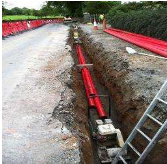
Image 2-1: Example of 110kV Underground Duct Installation
